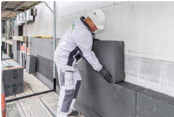
Insulation material installation, copyright BASF
